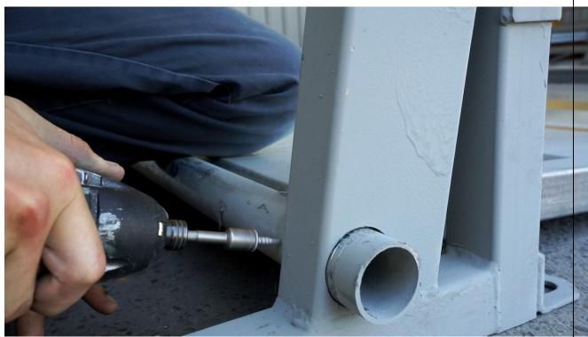
5. Attach metal end cap to base shaft as illustrated, secure with 3 tek screws as shown. Repeat on all 4 ends.
