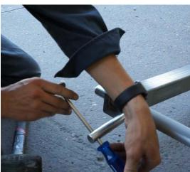
Screw the handle in place by hand and tighten using screwdriver as shown. Repeat for all 4 Slam Latches
