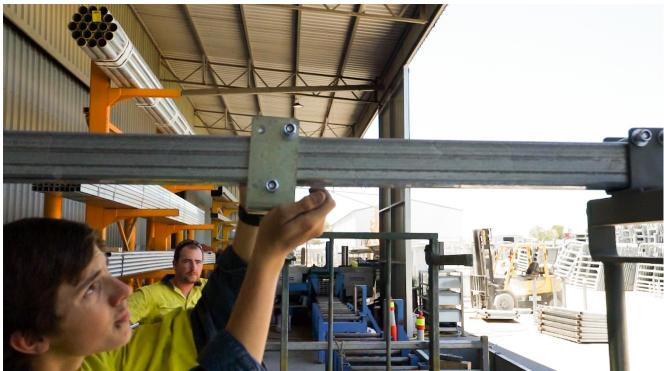
Attach the chain bracket, secure in place with bolts.
