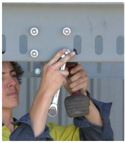
4. Ensure the gap between the frame and the side panel is even. Secure a tek screw on the inside of the base shaft as illustrated, repeat this on all 4 ends.
